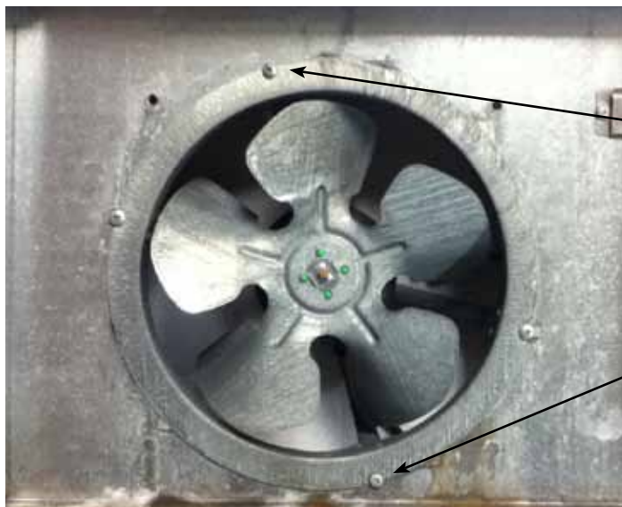
Figure 3. Completed installation of evaporator fan motor assembly.
