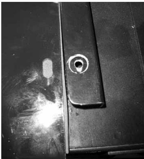
Figure 29. Align the holes in the trim with the holes in the top of the sign.
