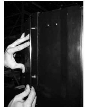
Figure 32. Once the holes have been drilled for all trim, install it as shown. Secure the trim with the 11/32" (9 mm) nuts from the kit.
