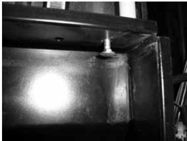
Figure 26. The carriage bolts (one on each side of the port) should hang loosely.
