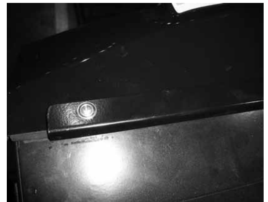
Figure 30. Trim and sign secured to door.
