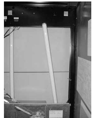
Figure 1. Angle the bulb to remove it from the door.
