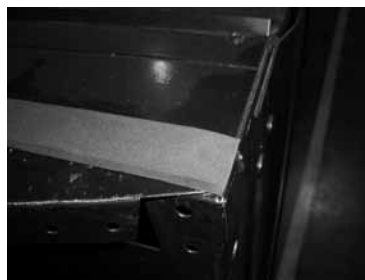
Figure 24. The foam strip should meet the right corner of the door.
