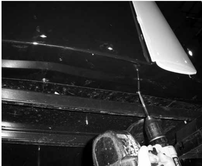
Figure 34. Secure the bottom of the door with two screws.
