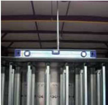
Leveling the front of the vender
